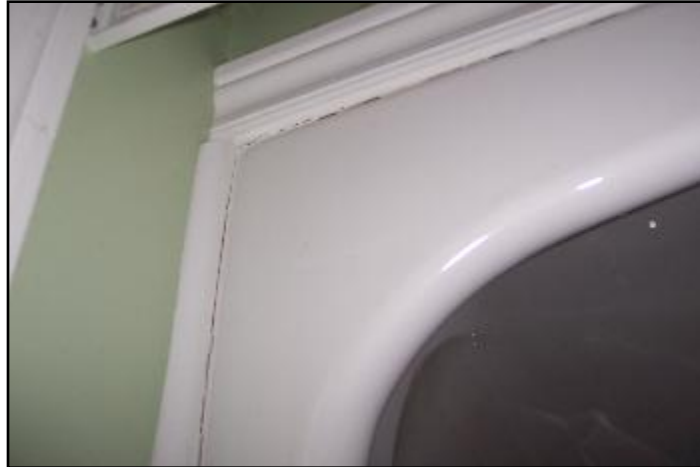
Caulking Deteriorated
