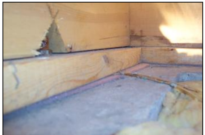
Same location, viewed from basement
