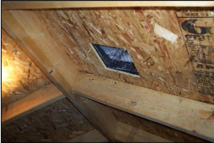
Roof Vent as seen from Attic
