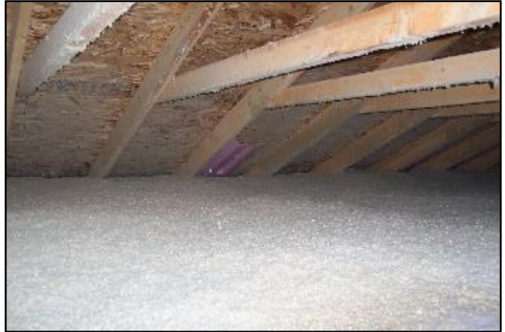
Soffit Vent Baffle as seen from Attic
