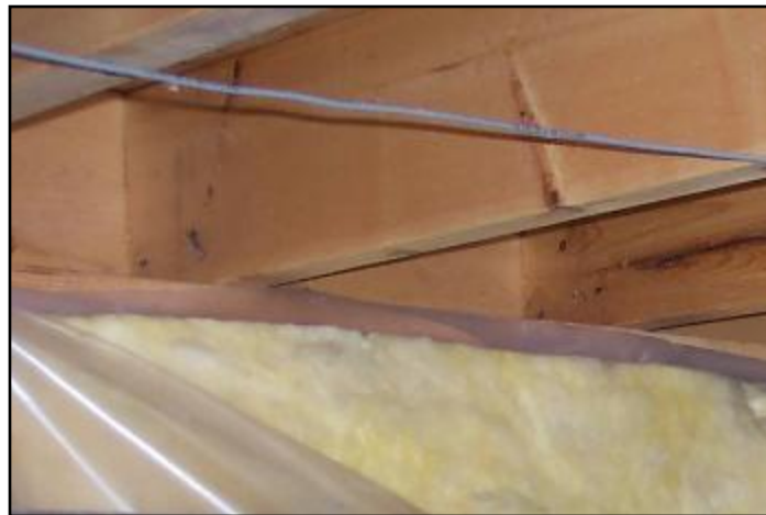
Insulation Stops at Top of Foundation Wall
